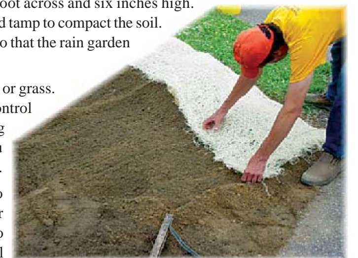
Erosion control matting made of coconut fiber is carefully placed along the berm to prevent erosion on the downhill side of the rain garden.
